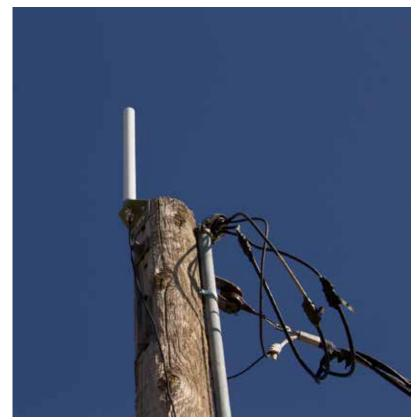
Antenna mounted on a wood power pole. Antenna cable is as far away from power wires as possible.
