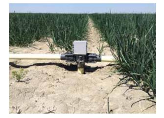
Here are examples of mounting the TWIGs on a stake or a pole. This method provides for going over the top the crop obstructions to get good line-of-sight. The wires from the solenoids must be extended to connect the TWIG wires.
